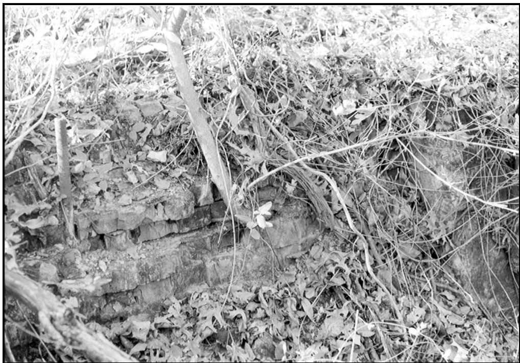
Figure 23. (TOP) View of the one of the engine mounts in Feature 8. The mounts are of composite construction (brick and poured-concrete). (BOTTOM) Brick was used as infill around the some the large bolts used to hold down the hoist engine (FRR November 2001).
