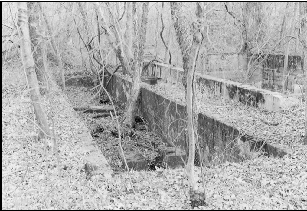
Figure 11. (TOP) View of the combination office and scale house (Fea. 1), looking southeast. (BOTTOM) View of the scale pit that is located on the north end of office/scale house. Railroad cars loaded with coal were weighed here before being moved onto the Illinois Central Railroad (FRR November 2001).
