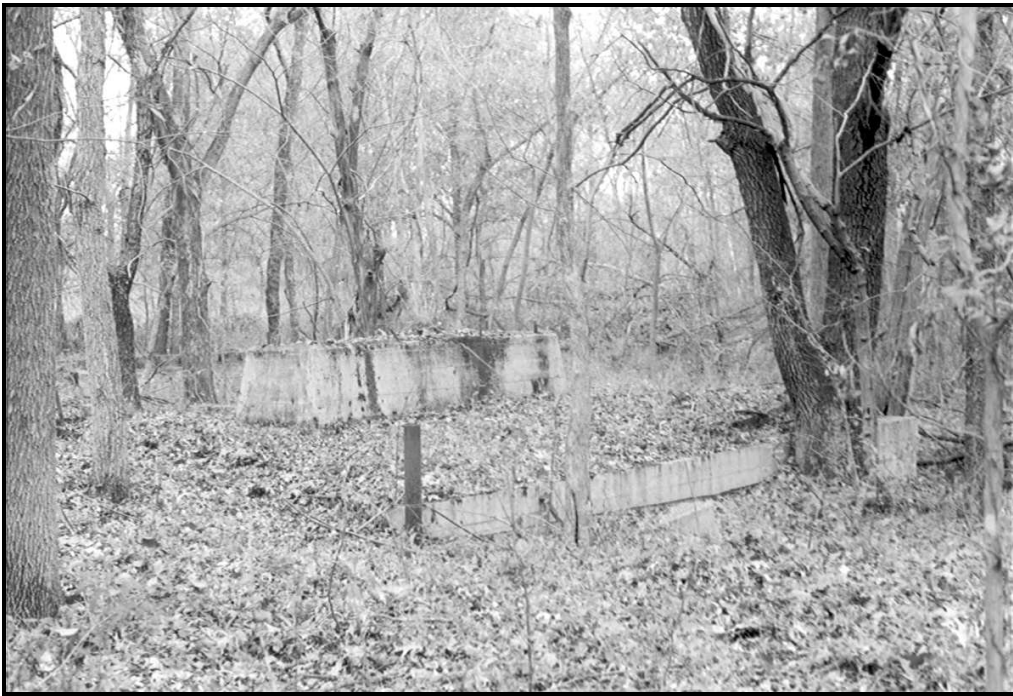
Figure 15. (TOP) View of the foundations remains of the fan house (Feature 4), looking northeast. The fan room (with pit) appears on the left, while the engine room (with mount) is to the right. The foundations of the office/scale house appear in the background. (BOTTOM) View of the southern side of the engine room of the fan house, looking northeast (FRR November 2001).
