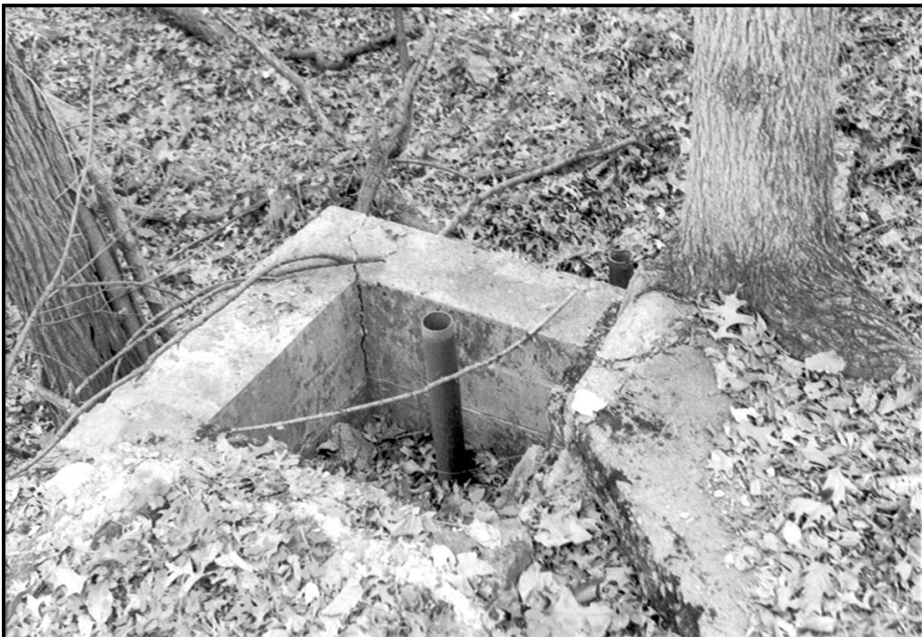
Figure 16. (TOP) View of the pit in the fan house in which the fan was located. This fan circulated clean air into the mine and drew out impure air in the process. (BOTTOM) View of the southeast corner of the fan house, showing the pit where water was piped into the building for the steam engine (FRR November 2001).
