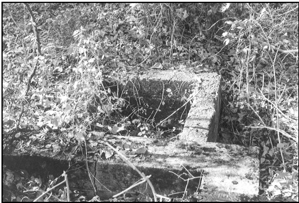
Figure 21. (TOP) Detail of the concrete drain that runs along the north side of Feature 6. (BOTTOM). This drain leads into a sump pit positioned off the northwest corner of the building (FRR November 2001).
